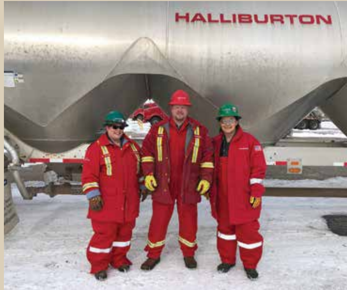
Noel (left) and Tonja (right) on Halliburton's cement operations job site with Aaron Hone (center).
